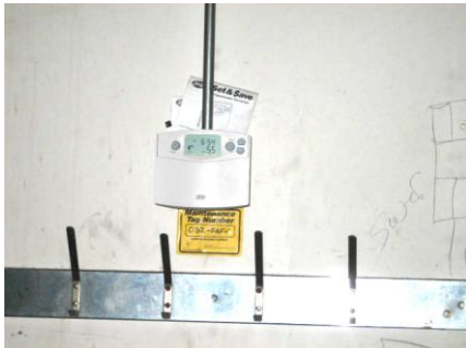
Programmable Thermostat installed in Water plant / Washeteria provides fuel savings
