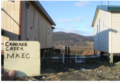
Heat Recovery lines were in the ground, stubbed-out and ready for hook-up
