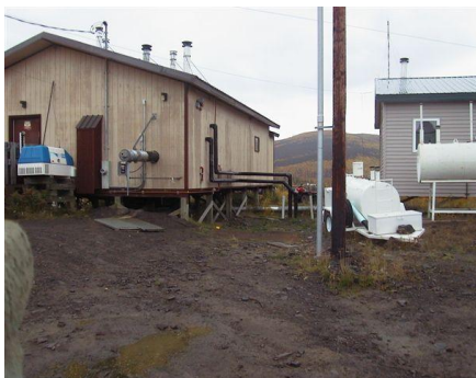
Completed heat recovery lines entering the Water Plant
